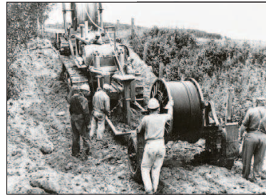
Cable is trenched into the ground to protect it from temperature problems and accidental cuts.
