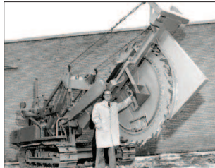
The industry has unique tools and equipment. This 1973 photo shows a Frost Wheel Trencher mounted on a trolley. It is used to lay fibre optic cable five feet below frozen ground.
